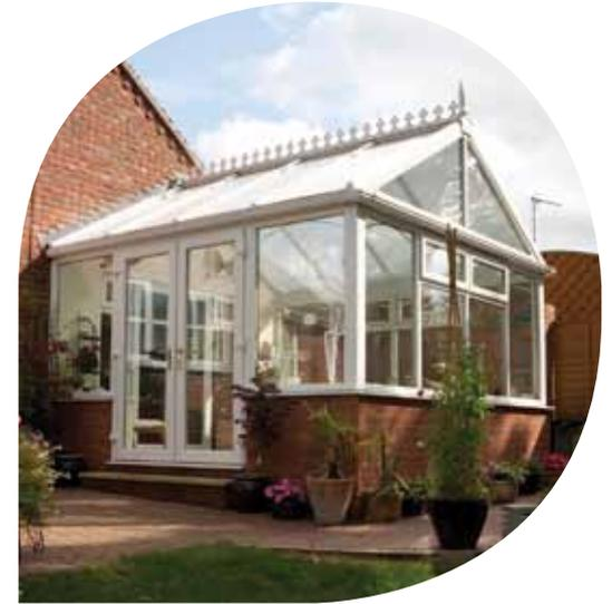
Gable style conservatories have two sloped roof sections ending in a vertical gable end, like many house designs. The Gable style of conservatory works extremely well with older properties, and can help to echo the style of the main building.
